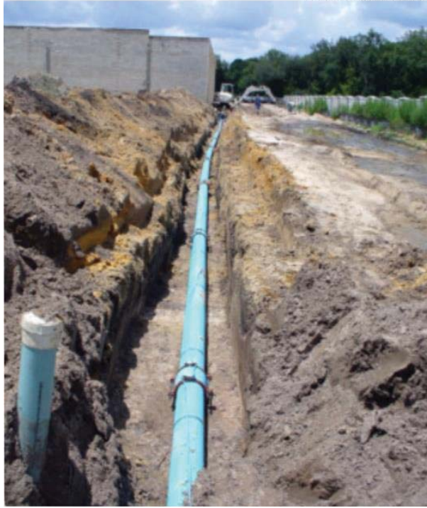
Figure 25. PVC pipeline installation.
