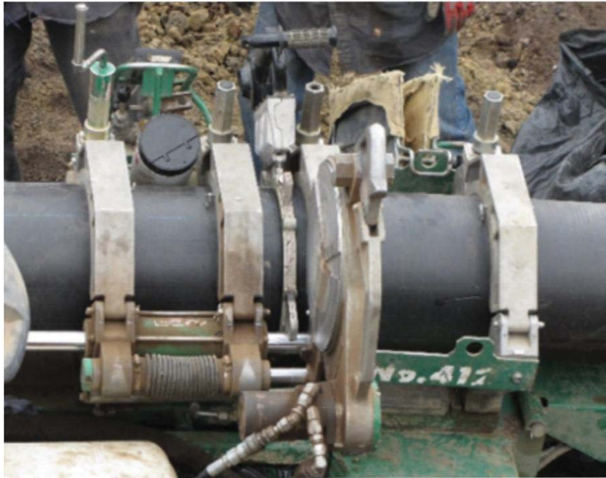
Figure 28. Thermal fusion joint.
