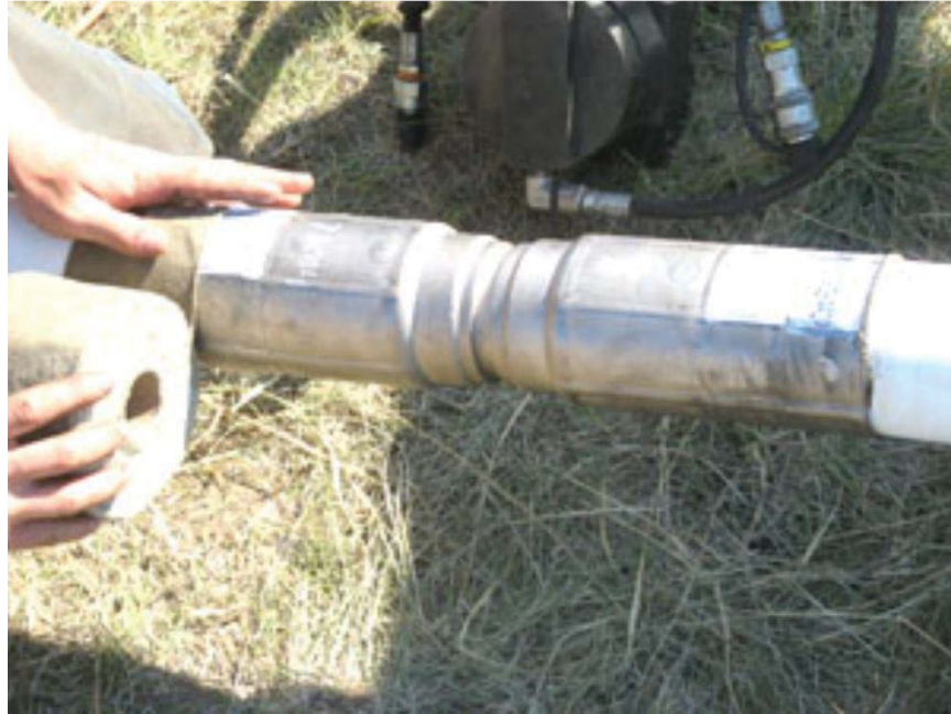
Figure 38. Flexpipe compression fitting.
