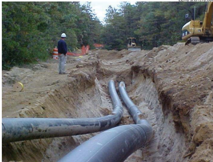
Figure 26. HDPE pipeline installation.
